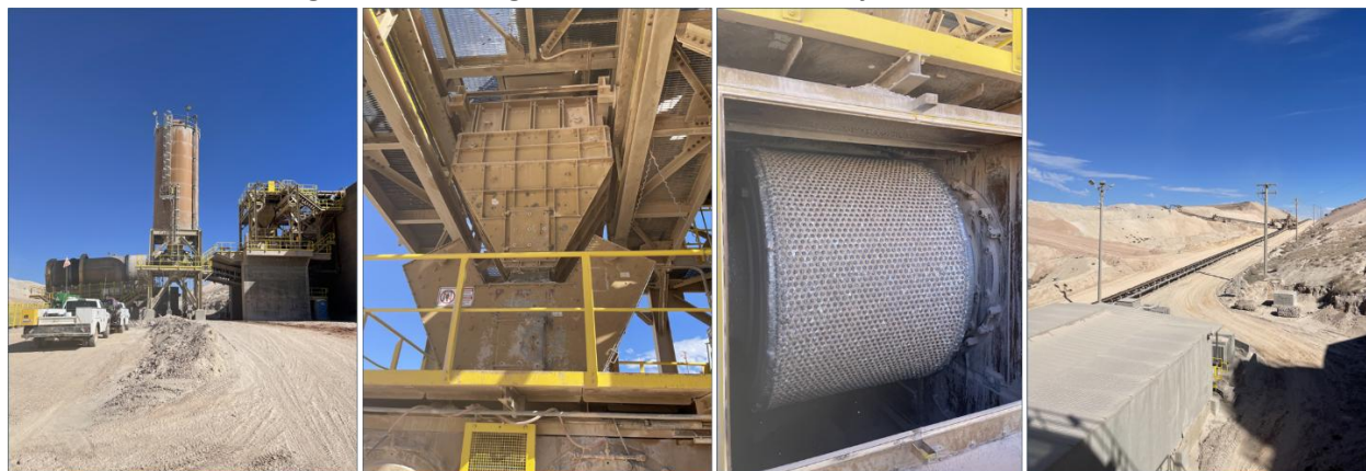
Figure 6: Crushing circuit, HPGR, and conveyer belt to stacker
